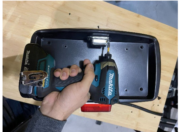
Fig. 9: Using a drill to unfasten the license plate light
